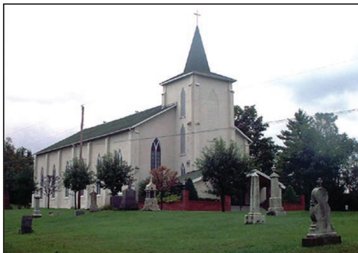
SAINT BARTHOLOMEW CHURCH, WILMORE
