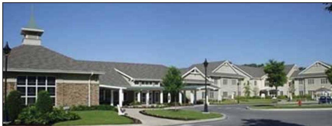
GARVEY MANOR AND OUR LADY OF THE ALLEGHENIES RESIDENCE
