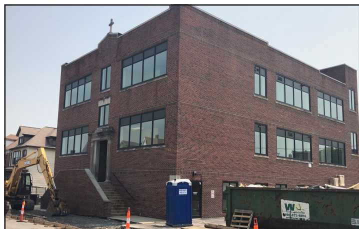
NEW PASTORAL CENTER: Exterior and interior work continued in early June at the former Our Lady of Lourdes School in Altoona. The building, to be called the Mary, Mother of the Church Pastoral Center, will house most diocesan offices and ministries.
